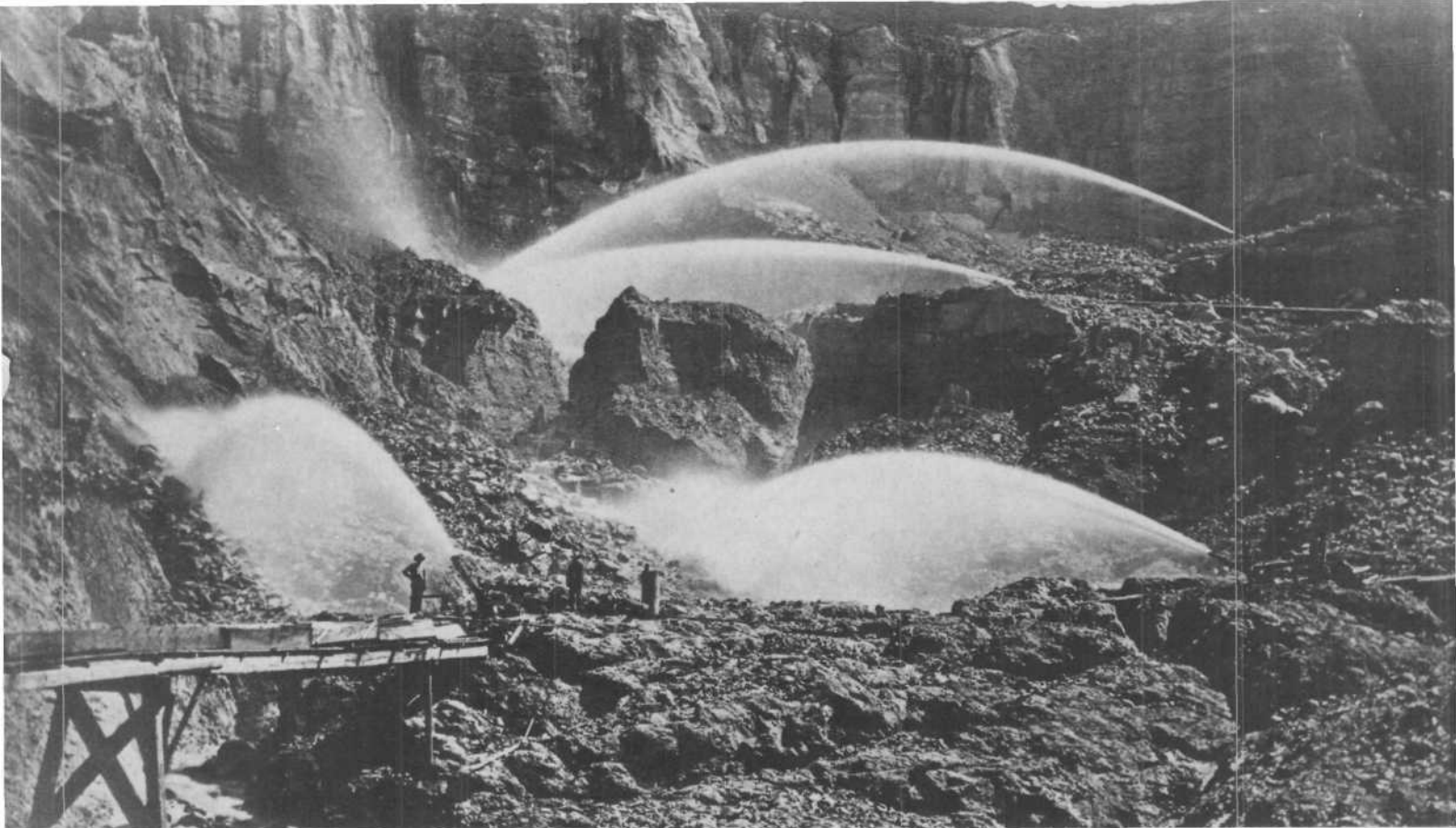
Hydraulic mining, North Bloomfield in Nevada County. Photo courtesy California State Library.
