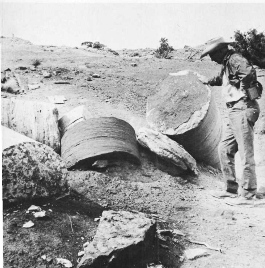
Lurt Knee examines the 36-inch cores which look like jelly rolls. Old mine entrance (right) shows ore-loading chute.
