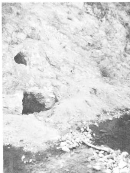
The stream was diverted through the mountain so alluvial deposits could be worked for gold.
