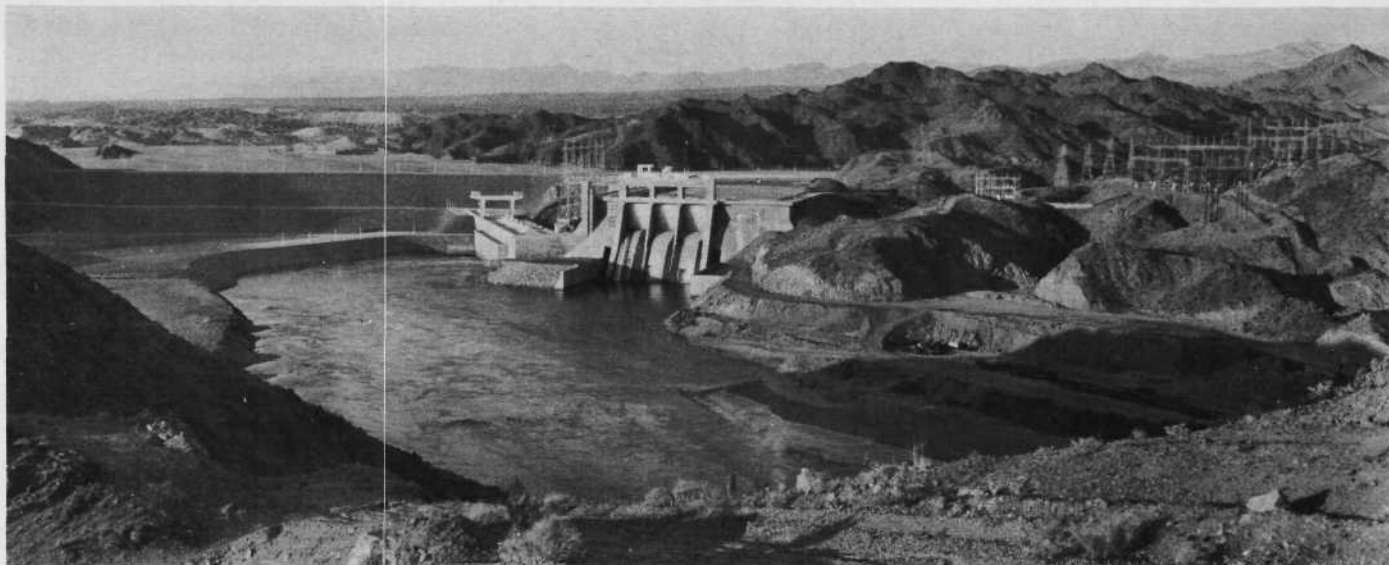
DAVIS DAM, LOOKING NORTH FROM THE NEVADA SIDE. CONCRETE SPILLWAY AND DAVIS POWERPLANT ARE IN CENTER OF PHOTO.
