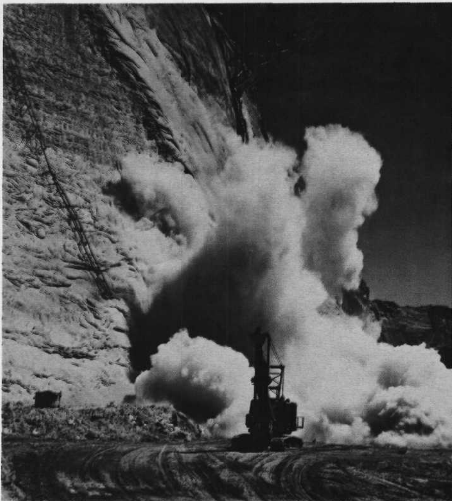
EXCAVATING FOR THE EAST KEYWAY
