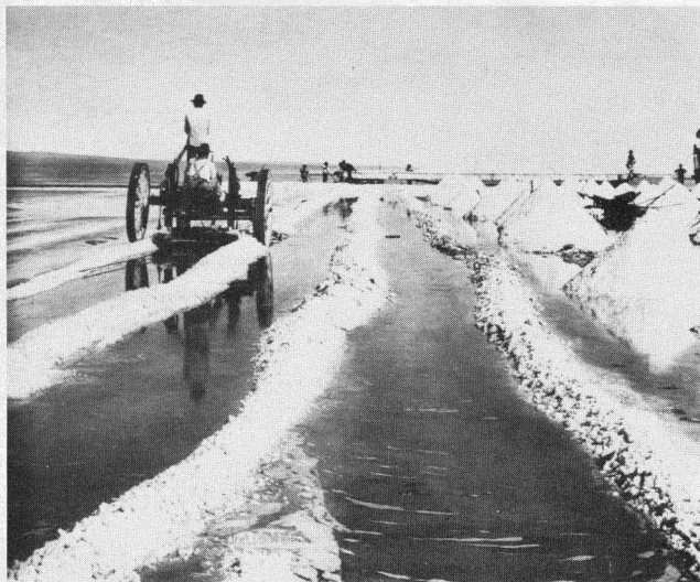
SALT MINE. Scraper, powered by donkey engine at end of long cable, harvests salt on the floor of Salton Sink in 1903—three years before flood waters created Salton Sea.
