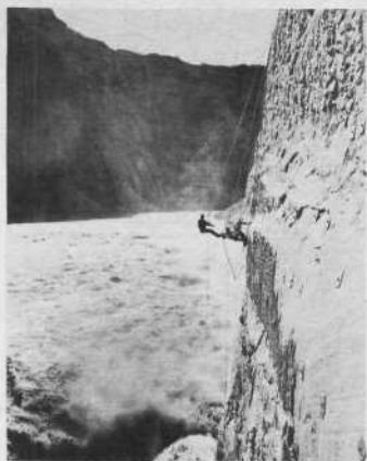
HIGSCALERS DRILL ON THE CANYON WALL JUST ABOVE THE RUSHING WATER
