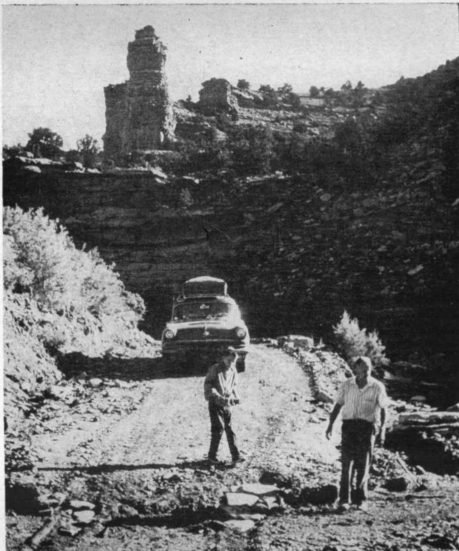
A washout on the Gateway Canyon road is filled-in with stones.
