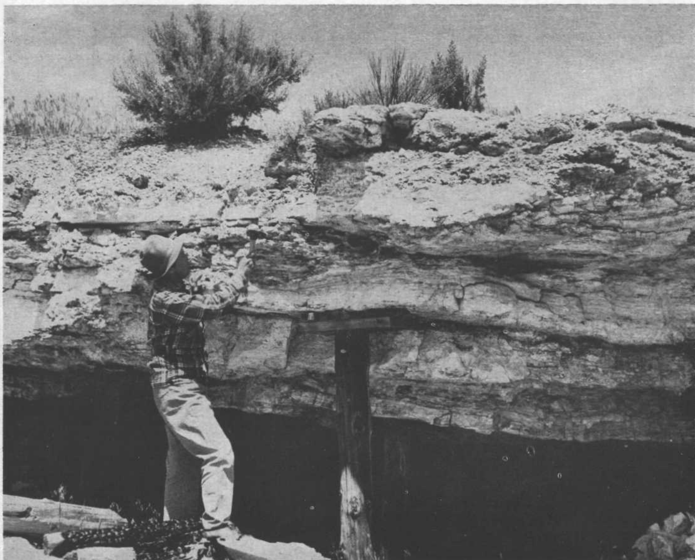
Author examining opalite ledges where miners "gophered" beneath the overburden to rich cinnabar ore. Old stulls still are in place.
