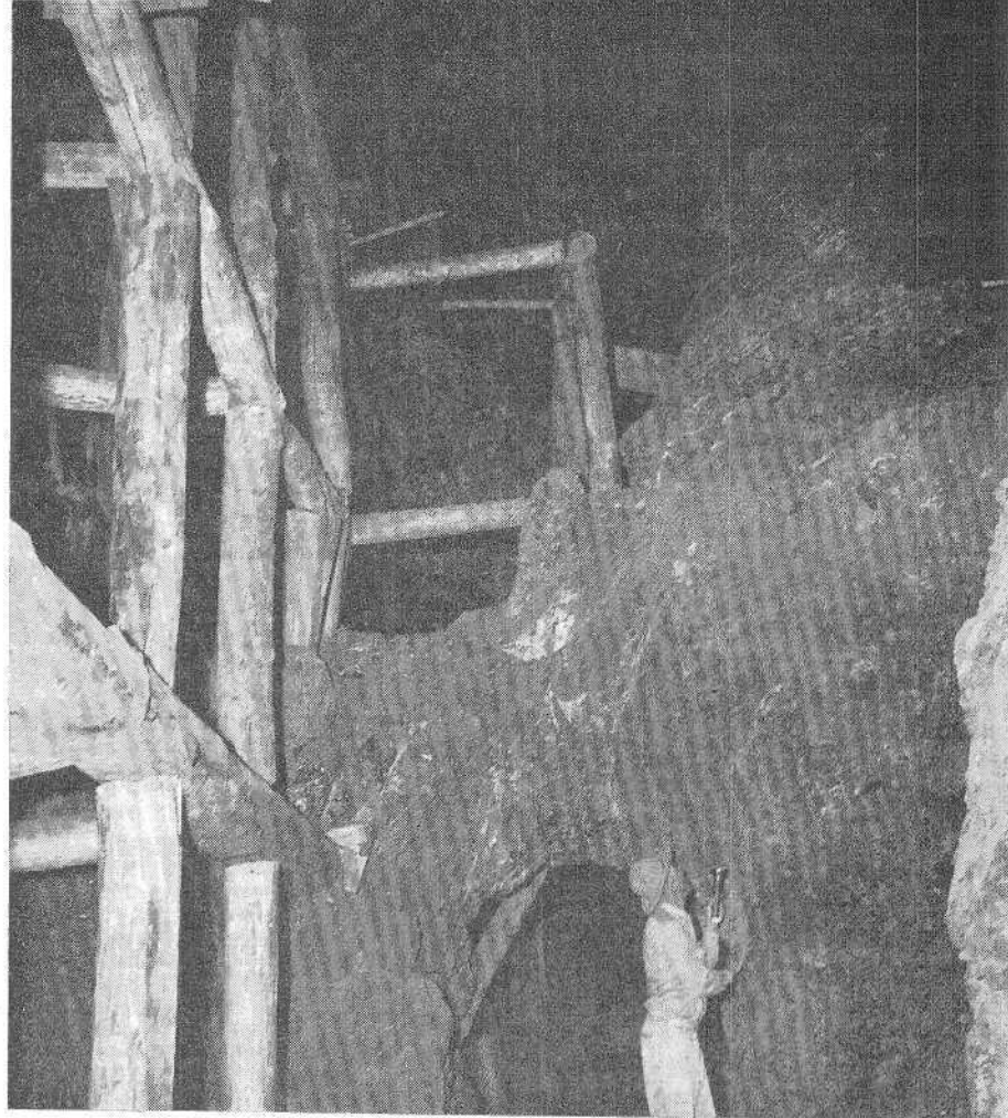
Ed Rochester, in one of the glory holes of the Clip mine, examines rich lead-silver ore left in a supporting pillar of rock. The huge cottonwood logs, left, were cut near the Colorado seven miles away, hauled to the mine and put in place nearly 75 years ago.
