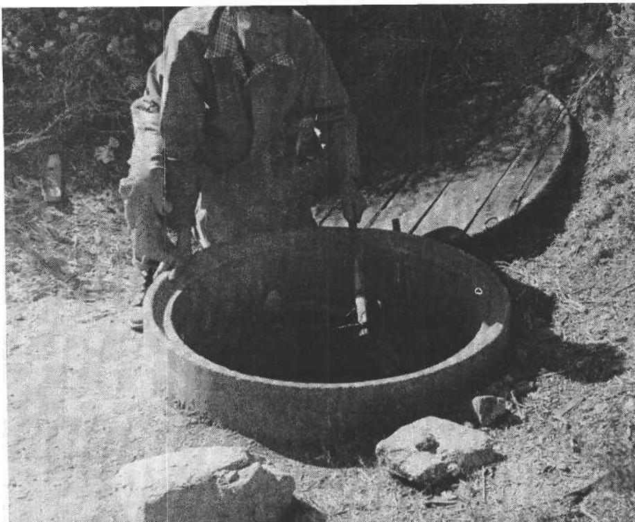
The author dips a drink from Yaqui Well. A section of concrete pipe serves as a casing for the well, and the wood cover keeps the water clean and pure.
