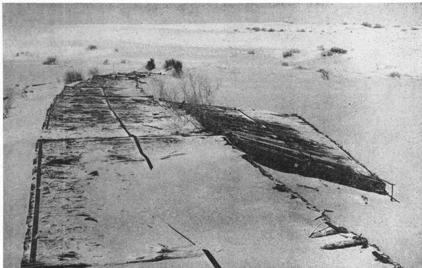
Wheeled vehicles first crossed the great dunes by means of a plank roadway laid on the sand and dug out and relaid after every storm. The roadway was so narrow that a strip for passing, plank at right, was provided every quarter mile or so.
