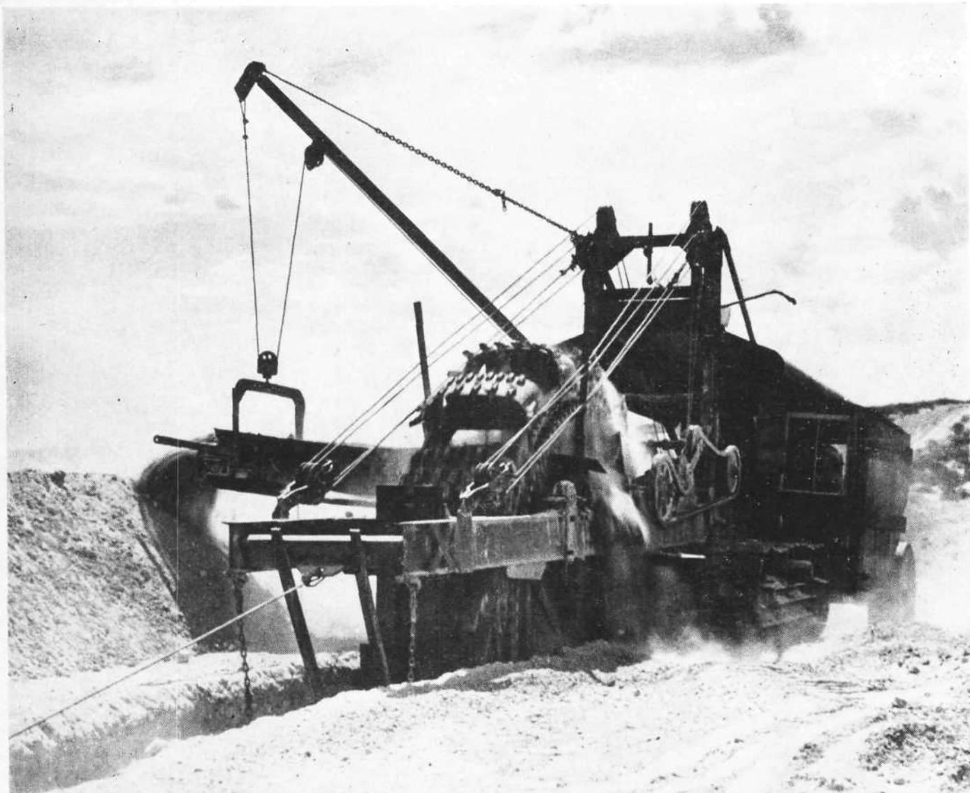
*Trenching machine of El Paso Natural Gas Company digs into Southwestern soil after trained archeologists have checked the ground for evidence of ancient civilizations and wave the go-ahead.*
