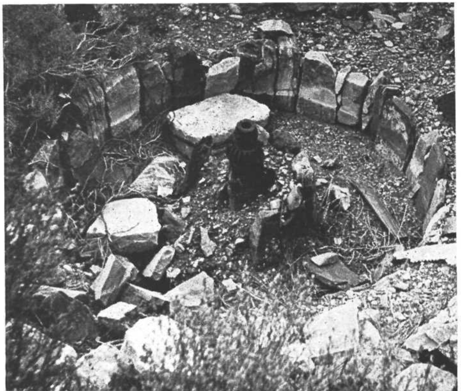
The upper arrastre in Johnson Canyon. Scour marks indicate the little mill saw heavy use. The drag-stone, its cable still attached, lies in the basin behind the pivot gear.
