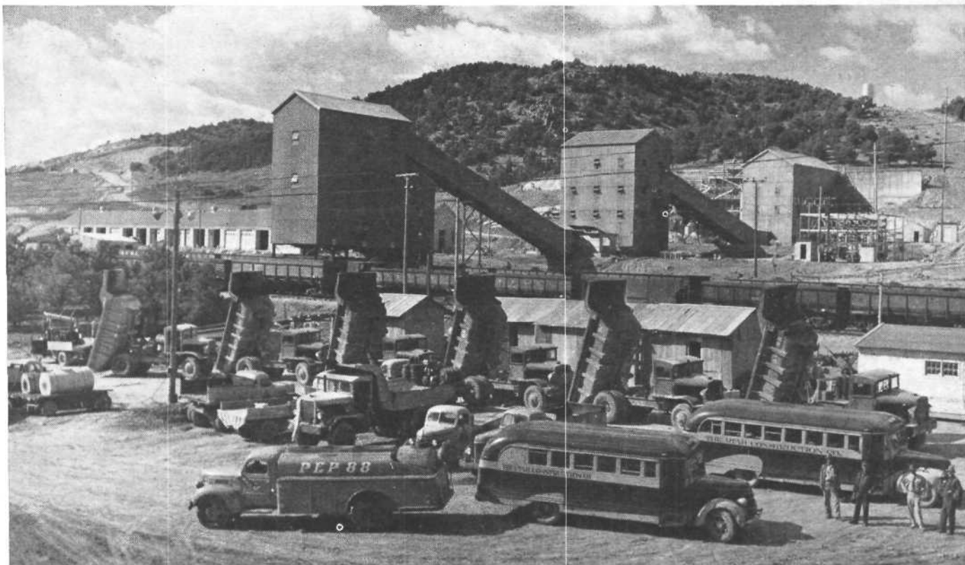
The large chunks of iron ore pass through crushing jaws of the reduction plants before loading into cars for a 200 mile trip to Geneva Steel Plant in Provo, Utah.
