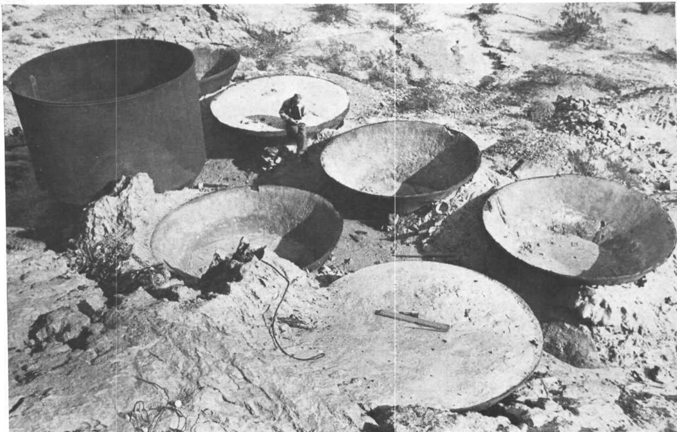
Settling pans, like giant crucibles, lie below the clayey silt dump of what may have been a flotation-type mill, no longer existing. The size of the pans may be judged by Jay Ransom, Sr., seated on a sediment filled pan.
