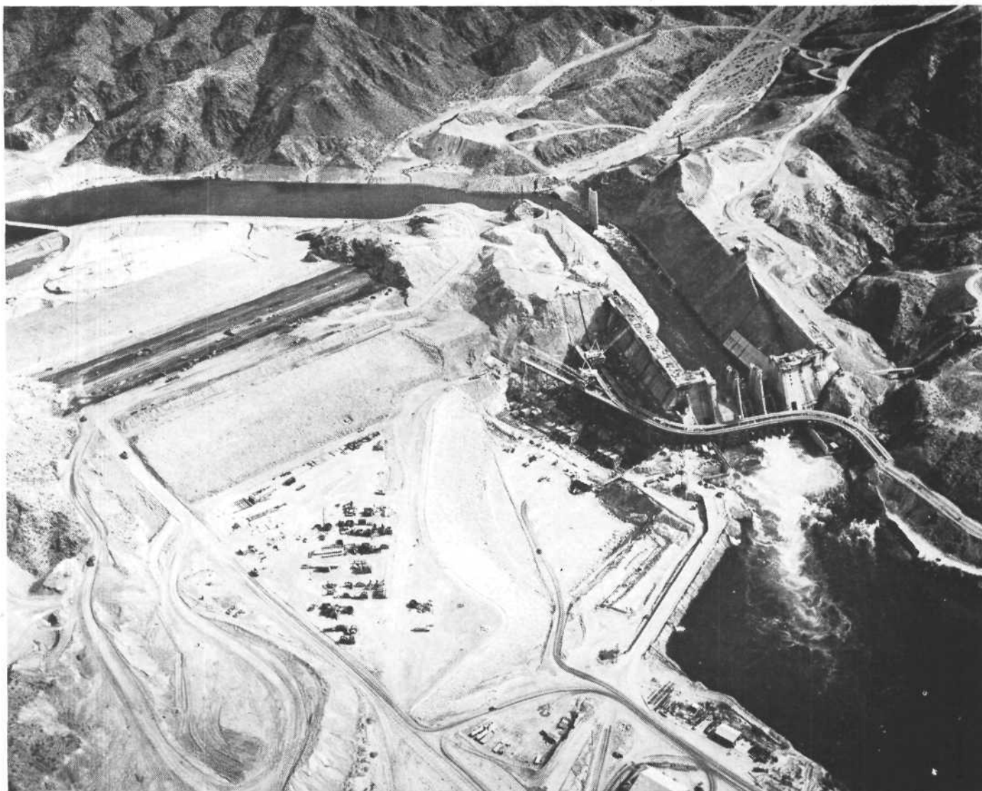
Aerial view of Davis Dam project. The dam is left center, blending so well with the coloring of the landscape as to be difficult to recognize. The spillway on the right is now being plugged with cement logs. Power plant is to the left of the gates. Lower cofferdam will be removed as soon as structure is completed.
