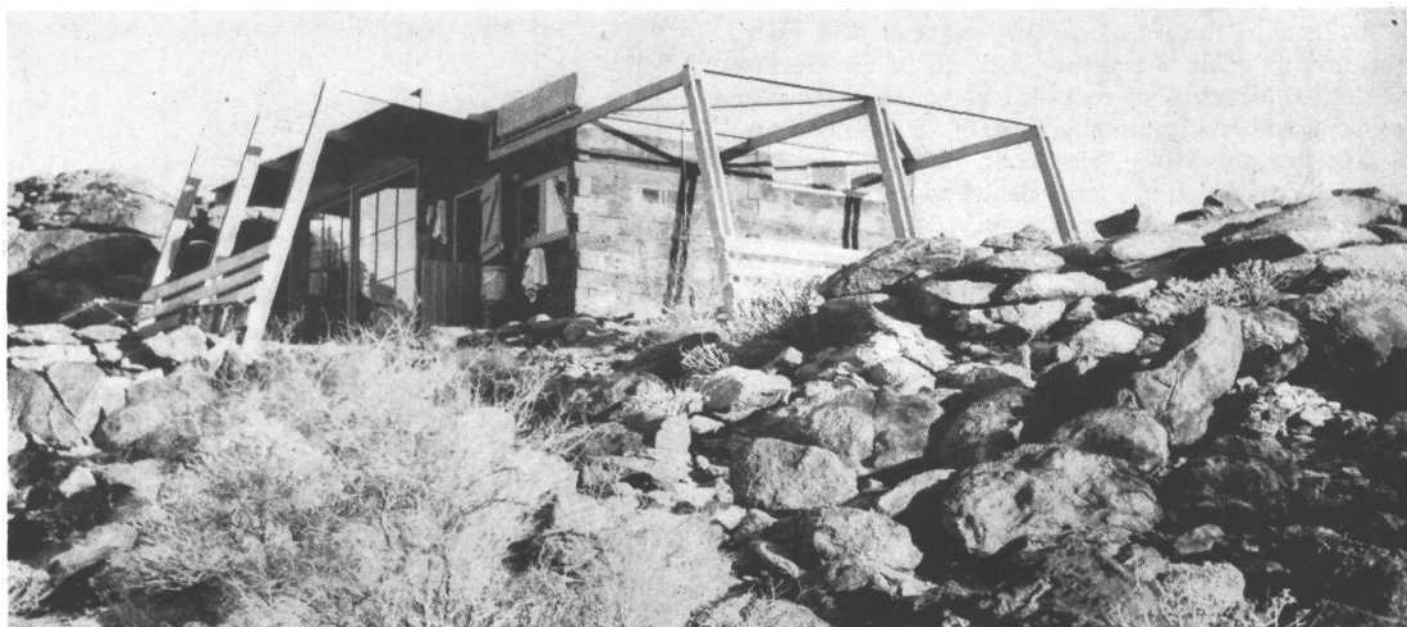
Built of railroad ties and country rock. The fins, anchored in cement, give added stability to the cabin.
