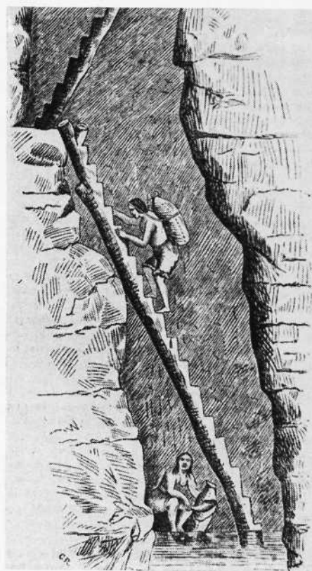
Sketch made in 1857 showing Mexican method of bailing water out of a mine shaft. Courtesy Arizona Pioneer's Historical Society
