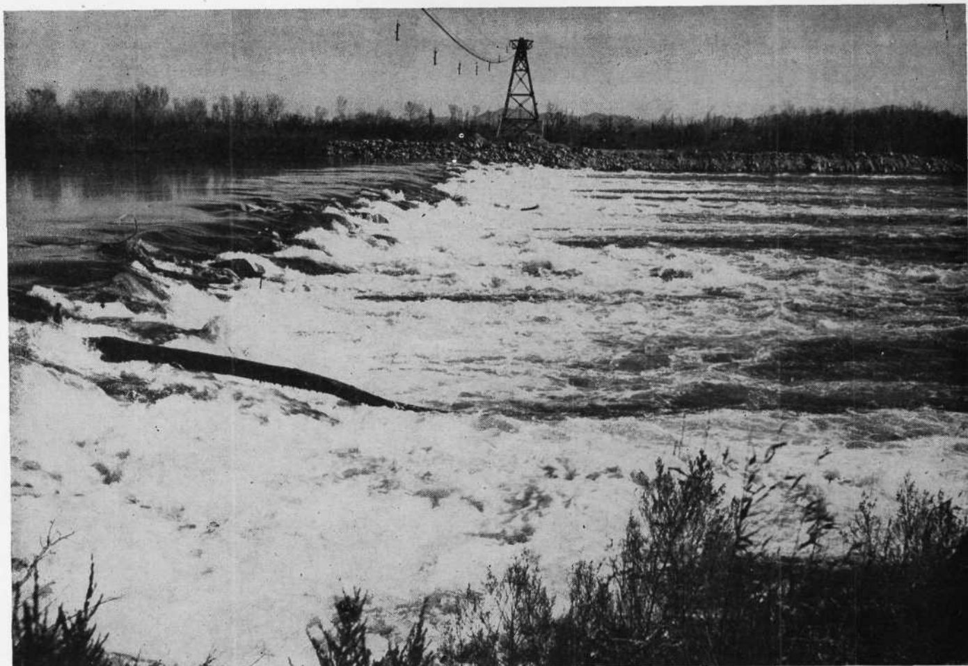
This rock weir raises the level of the Colorado and keeps water flowing into Palo Verde intake just above. In the old days the same purpose was served less effectively by jetties extending out from the Arizona shore on the far side of the picture.
