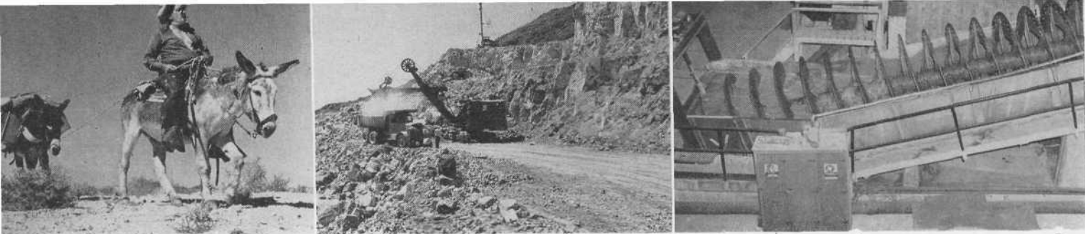
Left to right. 1—The prospector, daring desert heat and endless miles of hills and sand, deserves credit for locating the great deposits of magnesite from which magnesium is made. Photo by Truman D. Vencill. 2—Magnesite blasted out with dynamite is scooped up with big shovels, dumped into specially designed trucks which carry 20 tons of ore each, in steady stream to Gabbs plant, from where magnesium oxide and other concentrates are hauled to plant at Las Vegas, 334 miles away. 3—Ore is pulverized in a battery of ball mills (center), then moves to classifiers (foreground). Finer material flows out and is carried to the next operation.
