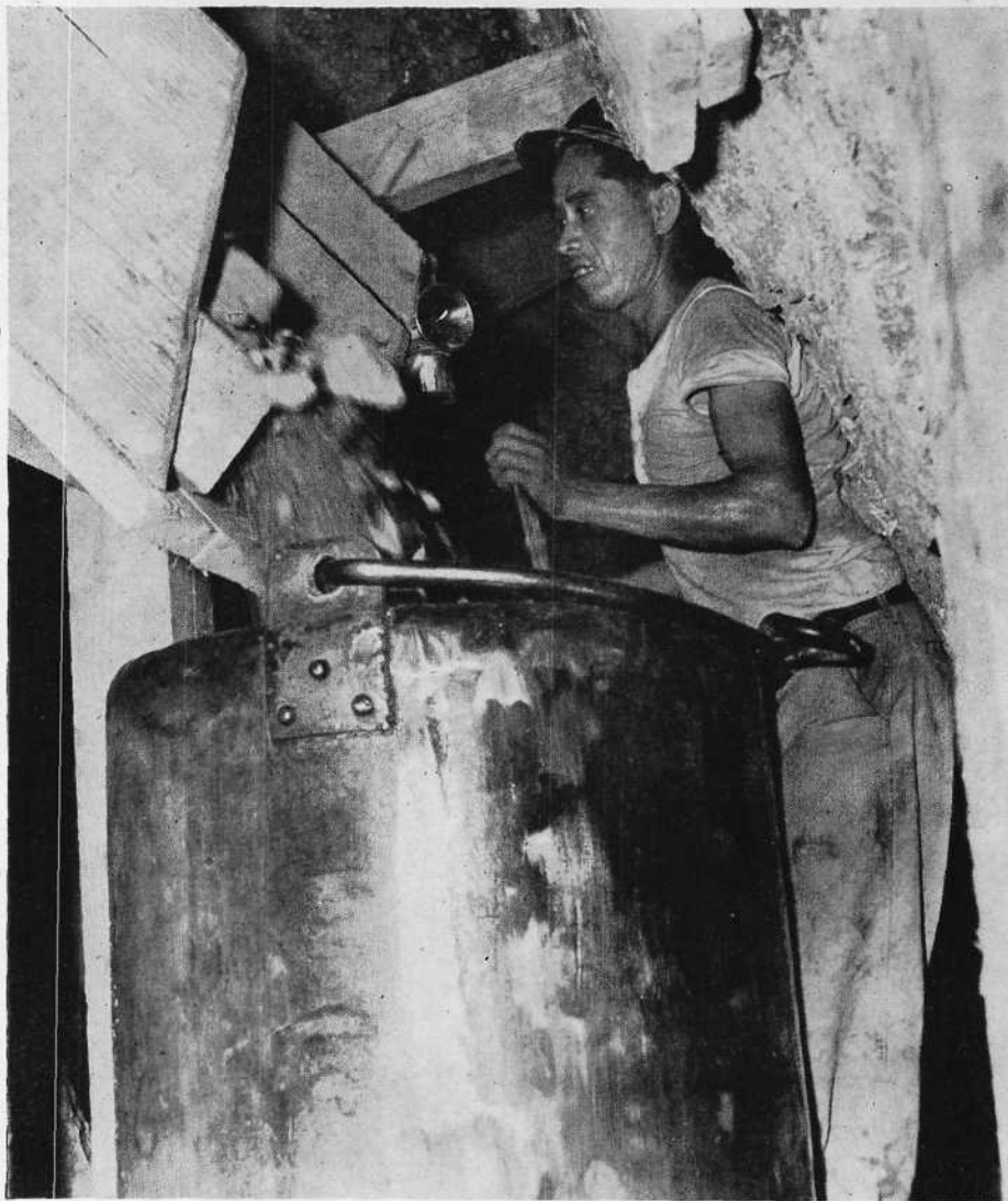
In this part of the shaft, ore is being "pulled" from a chute which leads to a stope above. When the bucket is filled, it is wheeled out to the main shaft where it is drawn to the surface.
