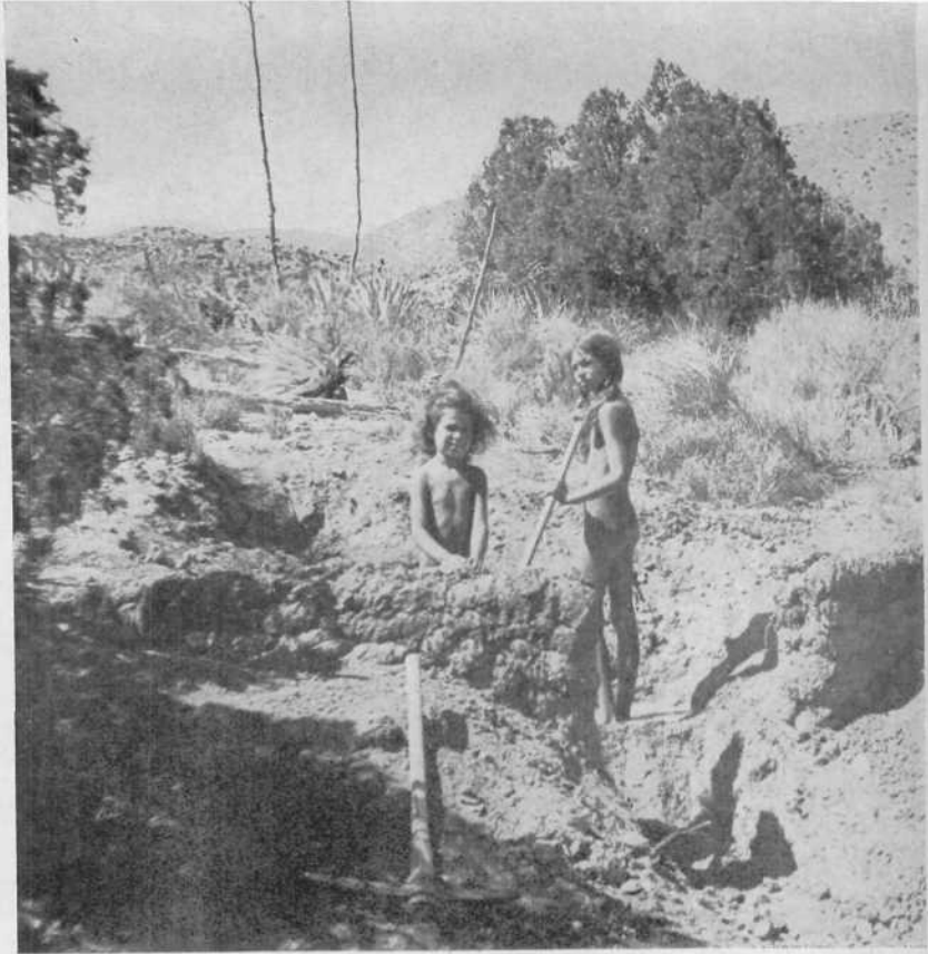
The storage house the Souths are building is a combination pit house and Navajo hogan. Rider tamps the mud while Rudyard plasters it on the wall.
