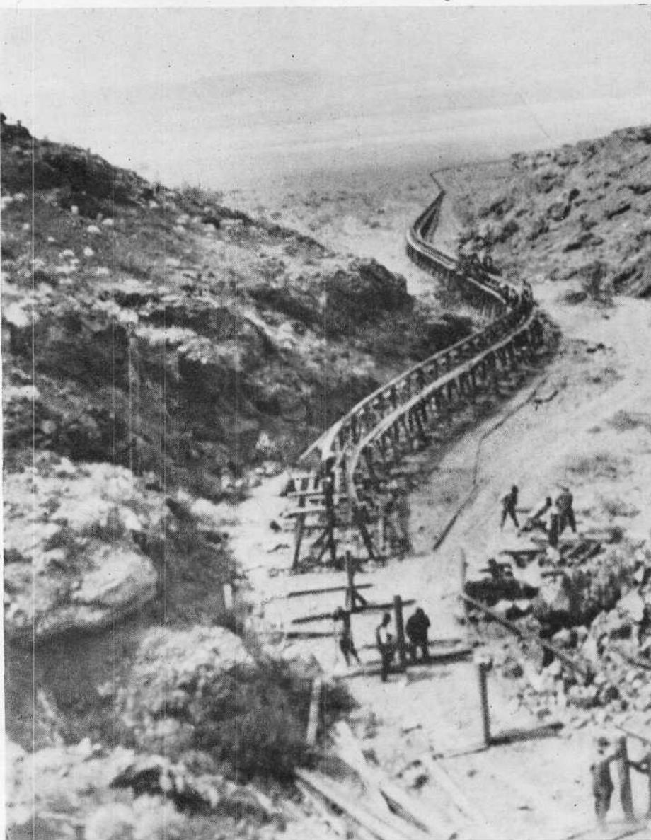
Like a great thousand legged worm the mono rail road crawls up through Layton canyon. View of construction work taken by unknown photographer. Photo loaned by V. V. LeRoy.
