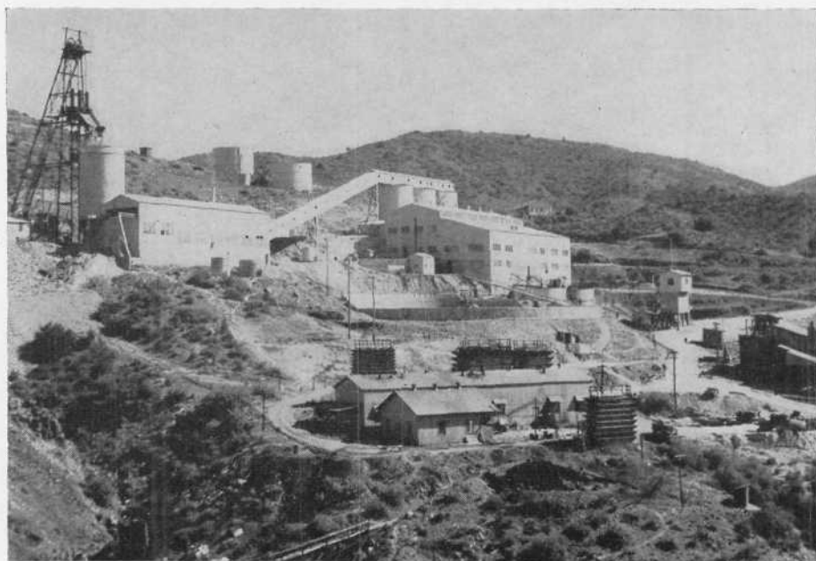
General view of the copper plant, looking east from an old mine dump. Left to right—Headframe, tank, crusher building, conveyor and mill. Water tanks on hill above mill and concrete settling tank below.
