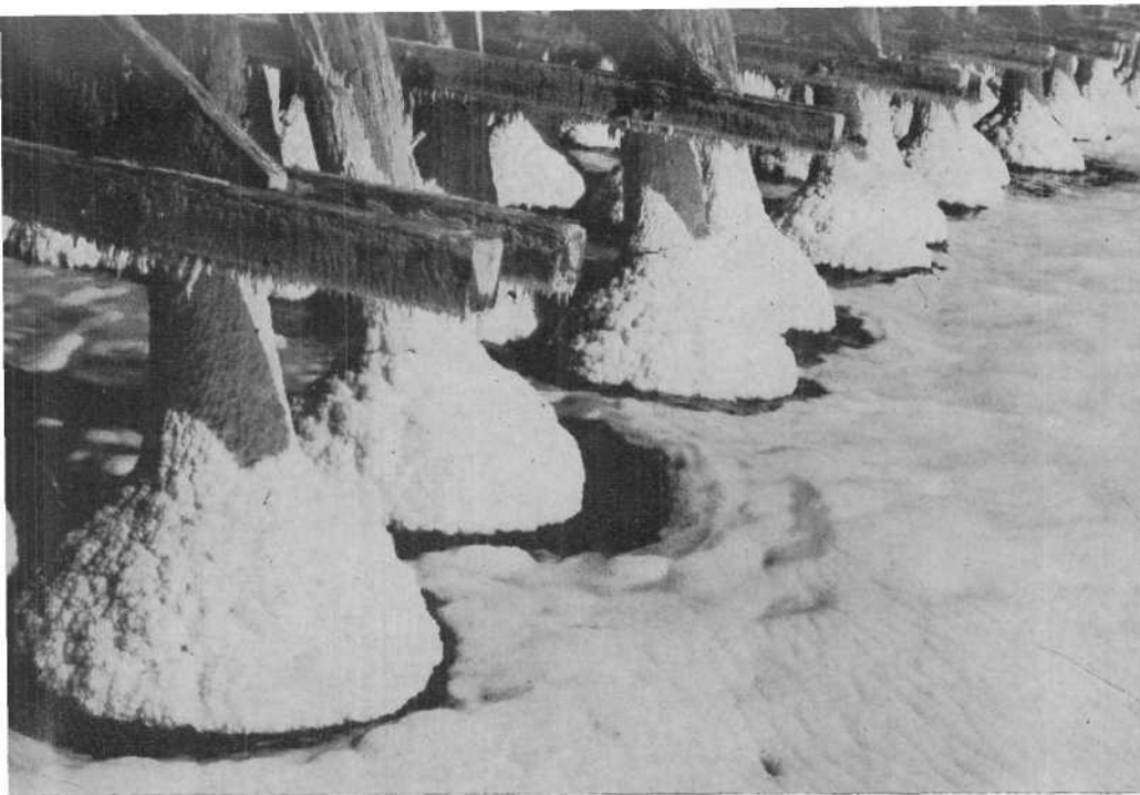
Accumulations of salt about the pilings of the railroad bridge across Great Salt Lake. Crystallization takes place only in late summer or early fall, when the salty water of the lake has reached a saturate solution due to excessive evaporation. Later in the season these crystals dissolve and the deposit changes chemically to a chalky white substance which crumbles easily.
