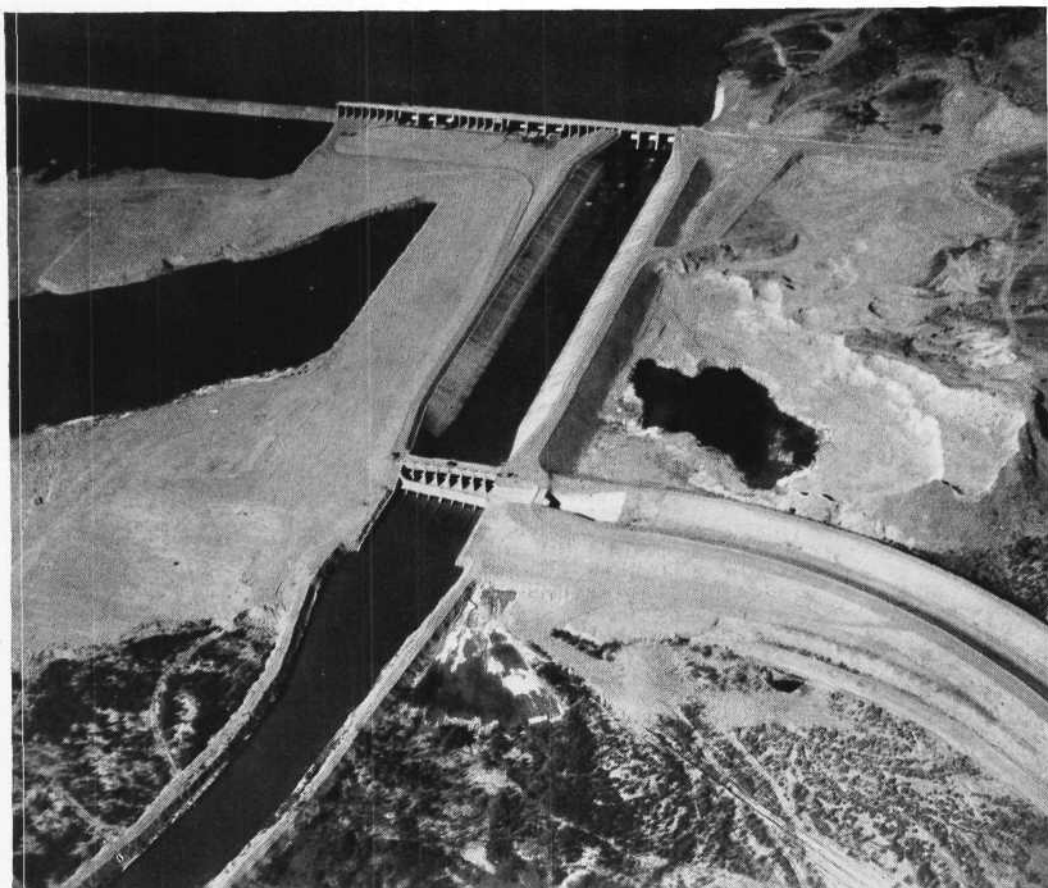
Imperial dam, where water from the Colorado river is to be diverted to the new Gila valley canal system. The basin below the dam is for de-silting the water. The Gila canal takes off to the right, in the center of the picture, and the sluing channel to the left.
