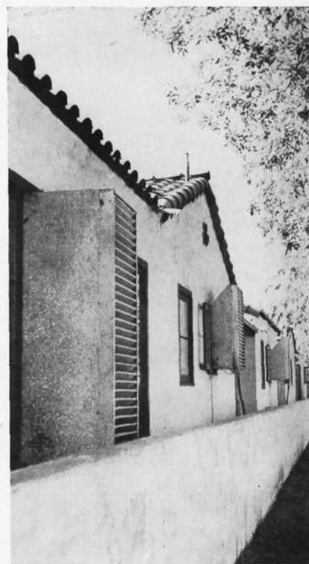
Many coolers are now equipped with louvers designed to hide the evaporative pads. The installations in this picture are on an auto court and show the improved appearance of current models.
