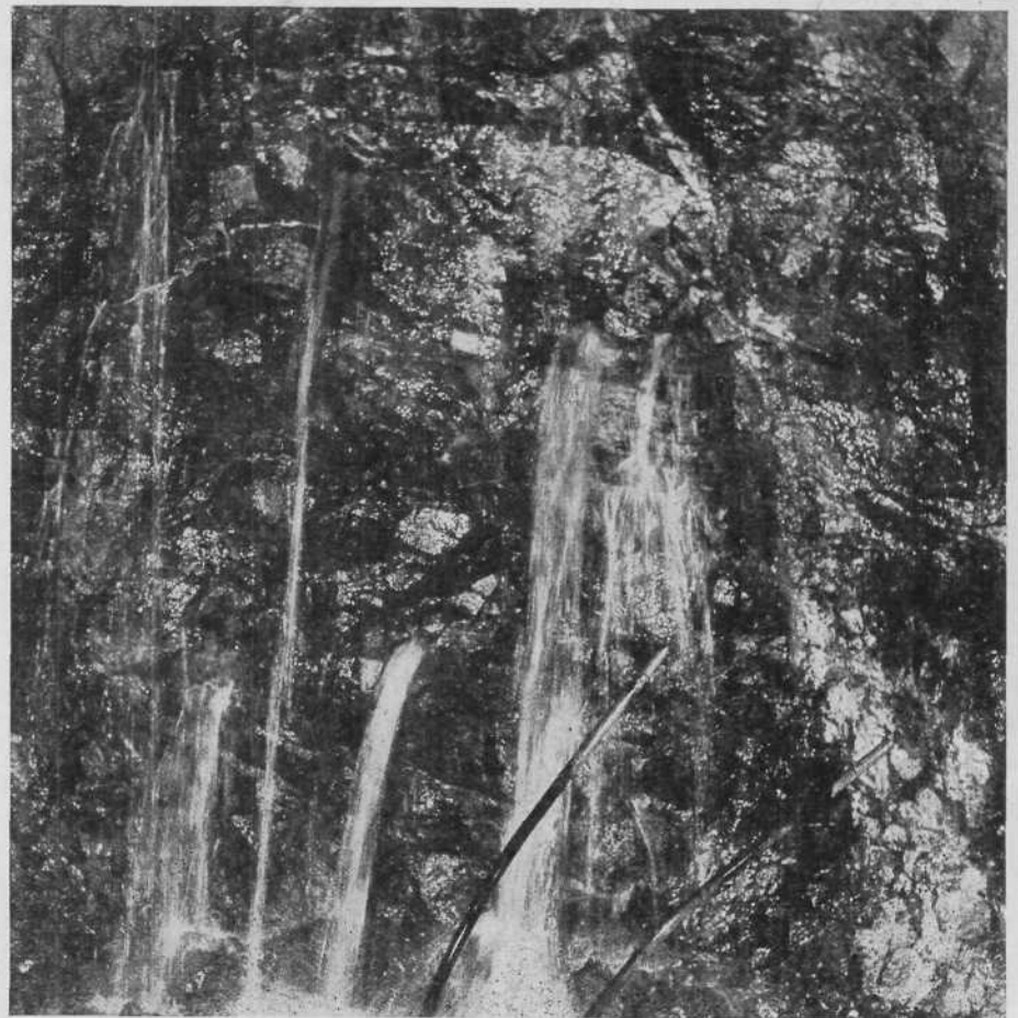
View of a small portion of a "Face" in San Jacinto tunnel, showing water pouring from fissures and drill-holes. Larger streams under tremendous pressure are sometimes opened when the face is blasted. Fox photo.
