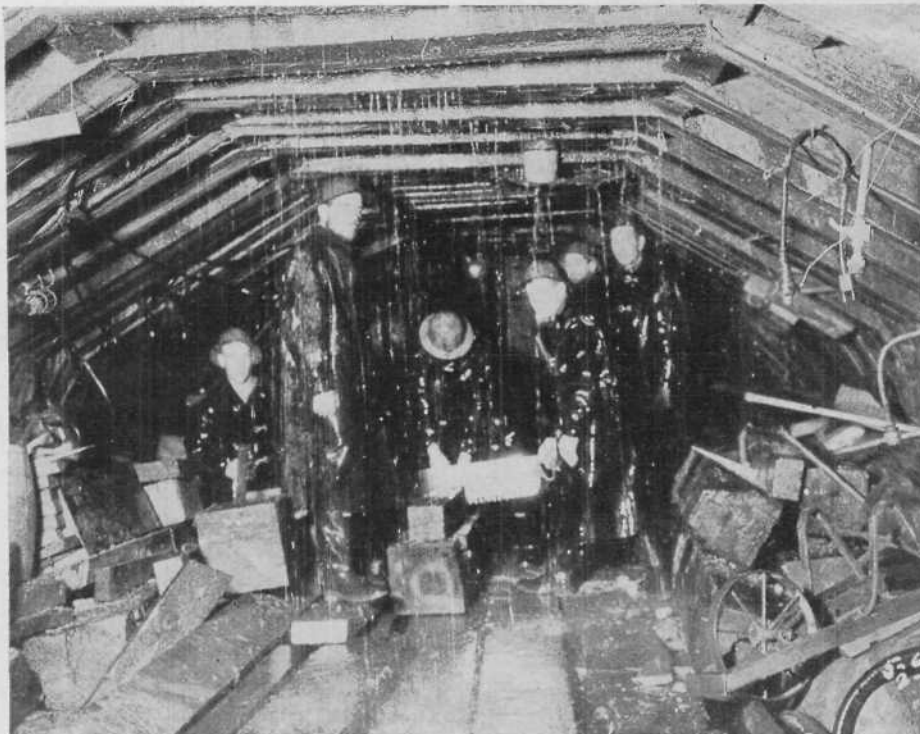
A tremendous amount of wood and steel is used in supporting the roofs and walls of the tunnel. The miners will work in the "rain" until the cement arch is completed. Fox photo.
