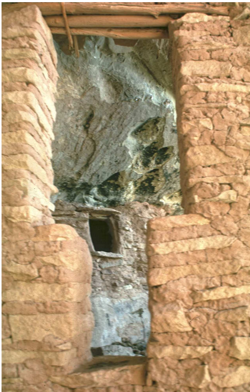
L-28. T-shaped doorway, with shaped masonry slabs, Upper Salt Creek Area, site 42SA21108.
