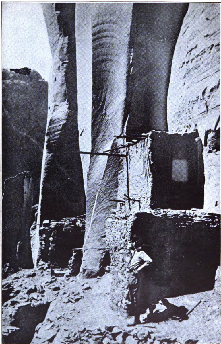
A near view of the westerly edge of the Betatakin Ruins. They are about one hundred to one hundred and twenty-five feet above the Canyon bottom. Note the cedar beams supporting the floor and roof.
