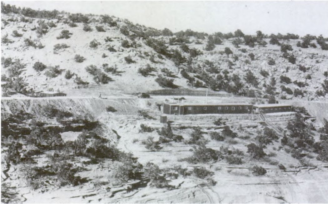
Figure 4.2. CCC camp NM-1-C at present site of Monument Canyon Trail parking area. Colorado National Monument Museum and Archive Collection.
