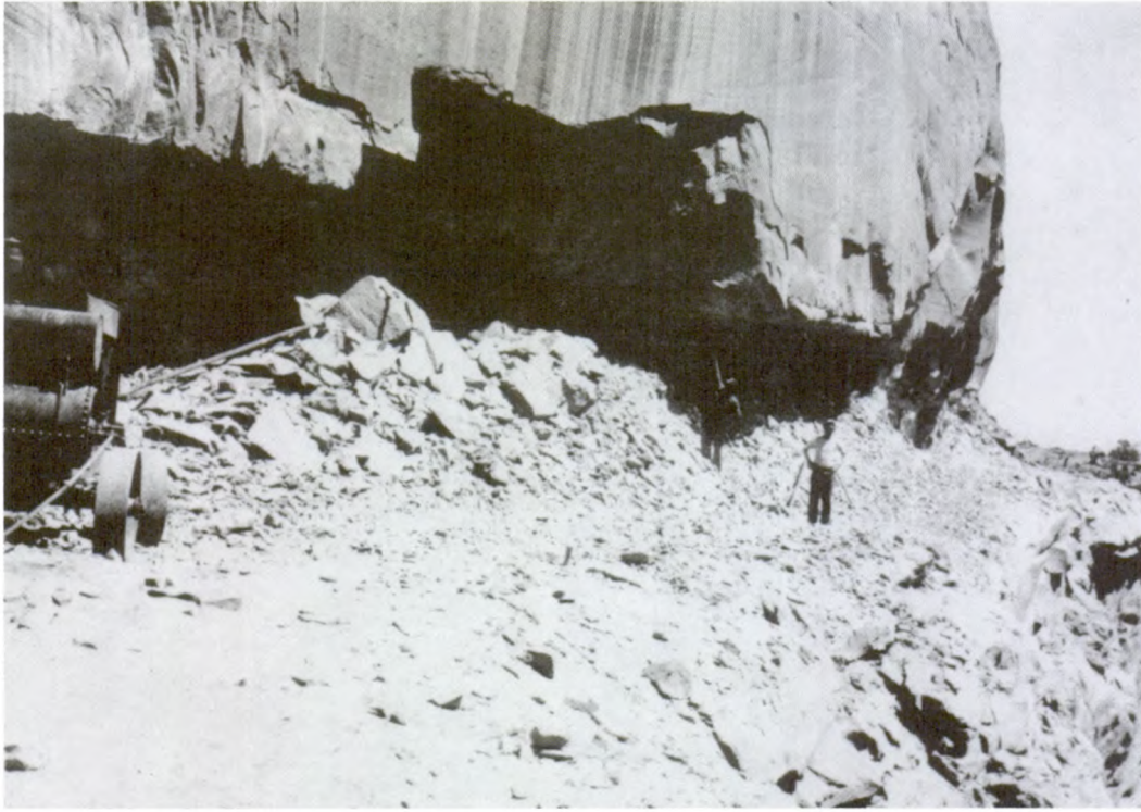
Figure 4.8. Half-Tunnel site after the December 12, 1933 accident. Colorado National Monument Museum and Archive Collection.
