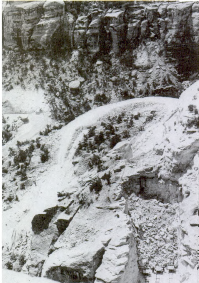
Figure 4.4. View from cliff above the south portal of tunnel #3 (bottom right) and east side road and switchbacks. Colorado National Monument Museum and Archive Collection. ▶ ▶ ▶
