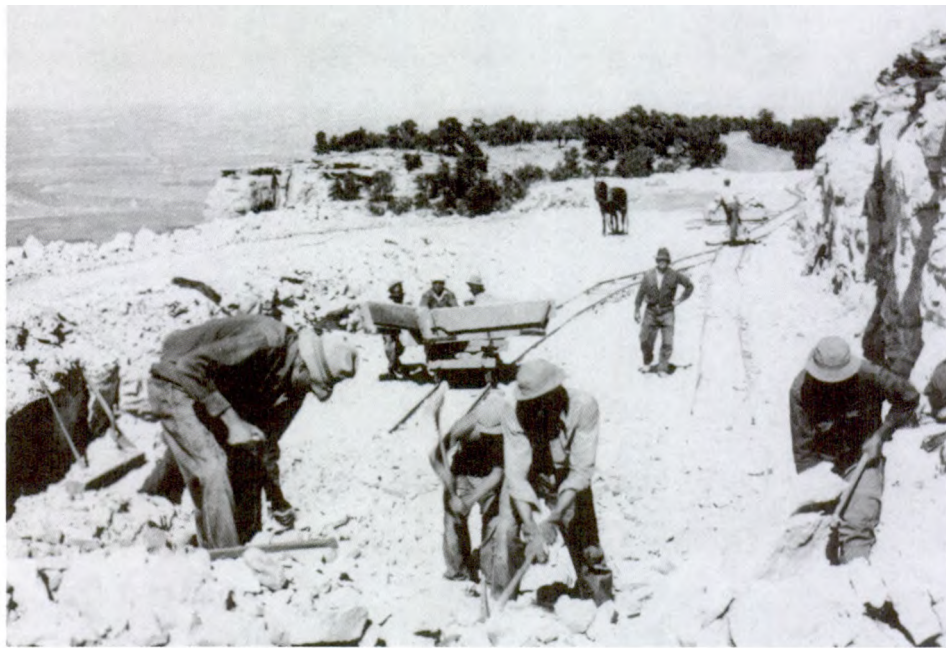
Figure 4.5. Men working at Cold Shivers Point on east Rim Rock Drive. Most of the work on the road was done by hand. Colorado National Monument Museum and Archive Collection.
